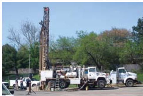
Well driller inserts one of 65 vertical ground loops.
