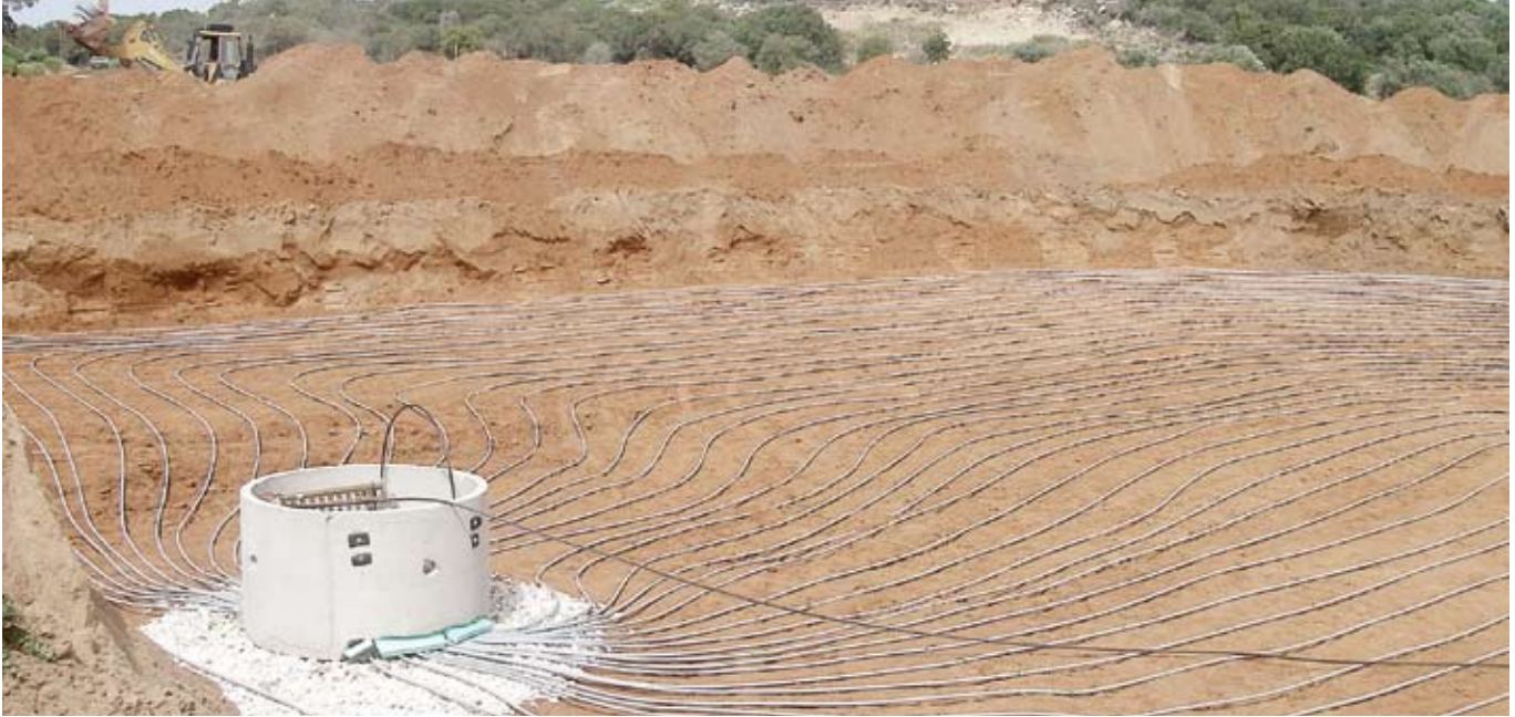
RAUGEO Collect horizontal ground loops connect to geothermal manifold in vault.
