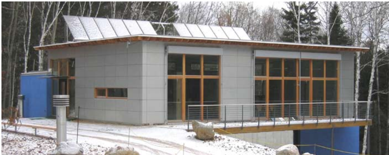
Many REHAU systems contribute to the outstanding energy performance of the BioHaus: ground-air heat exchange, solar thermal hot water, geothermal ground loop heat exchange as the energy source for radiant heating, and high performance vinyl tilt-turn windows.
